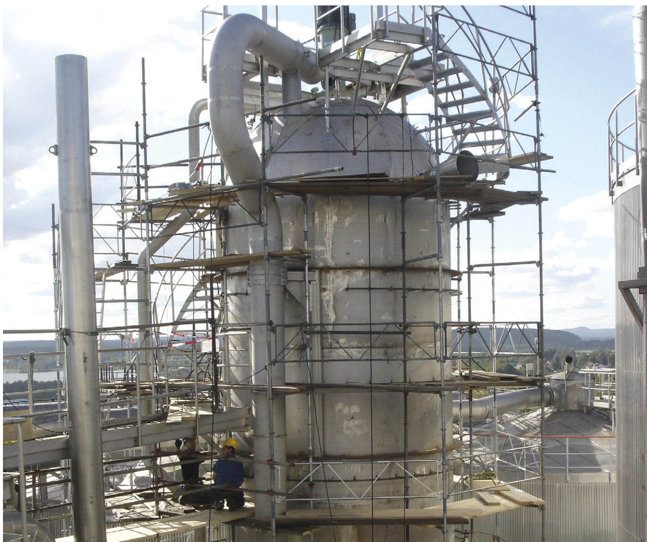
Figure 2. Hydrogen peroxide reactor in Forta LDX 2101 under construction, Smurfit Kappa, Piteå, Sweden. The reactor is 32 m high and 4 m in diameter
