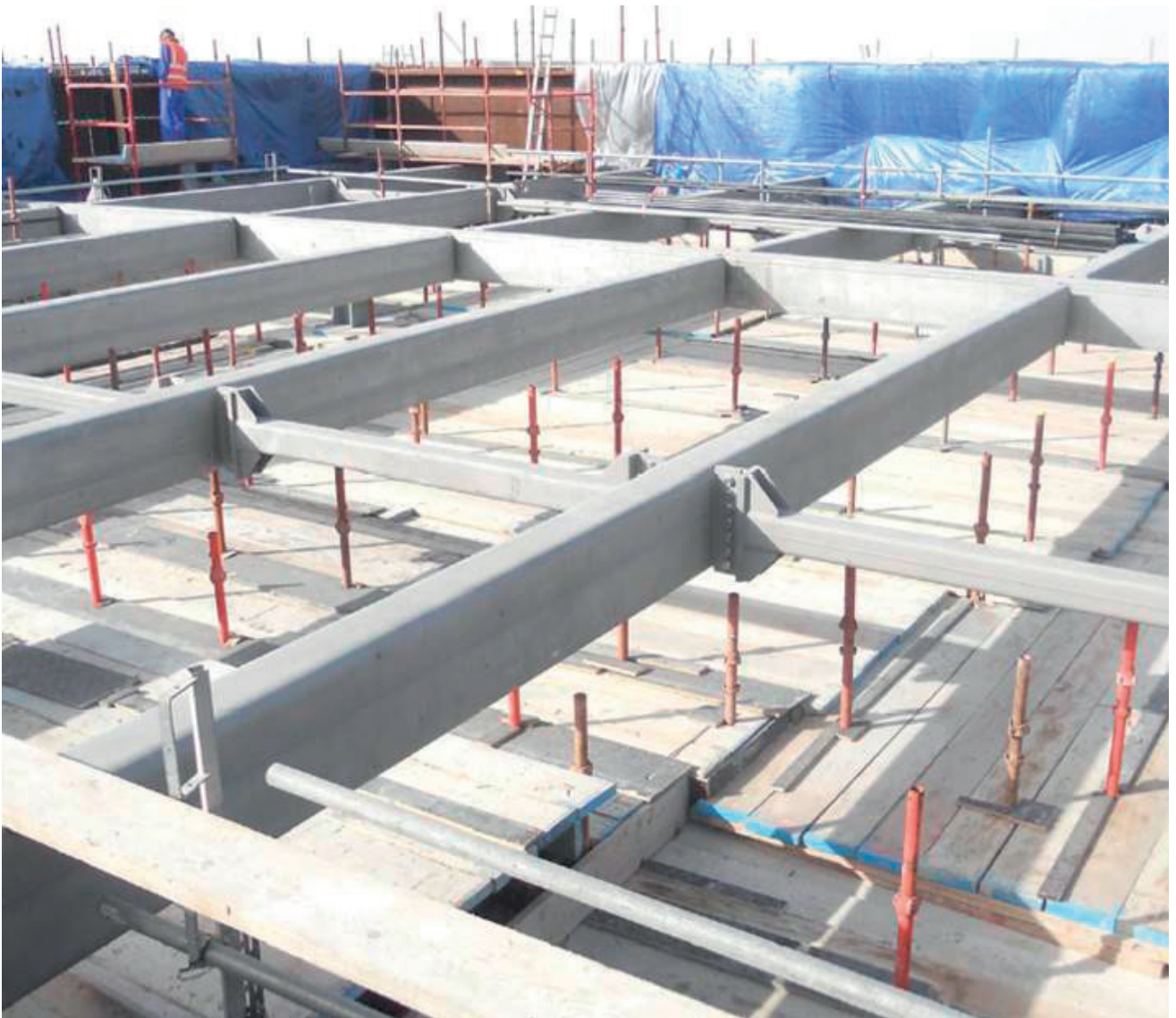
Figure 2 Detail of beam structure for the Qatar Foundation New Headquarters. Beams in grade Forta DX 2205. In total 170 tons of structural sections; 179 hollow sections in 17 different dimensions and 35 different L-profiles. Picture courtesy of Astad project management.
