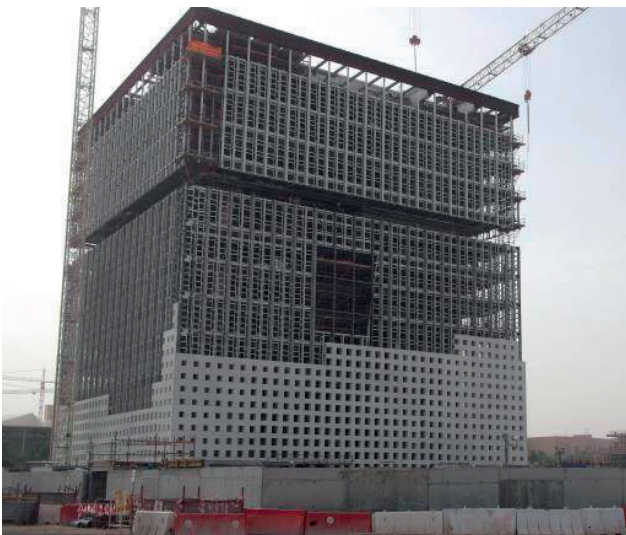
Figure 2 Detail of beam structure for the Qatar Foundation New Headquarters. Beams in grade Forta DX 2205. In total 170 tons of structural sections; 179 hollow sections in 17 different dimensions and 35 different L-profiles. Picture courtesy of Astad project management.
