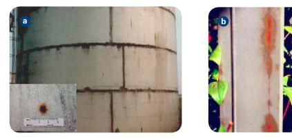
Stress corrosion cracking (SCC) is normally not a problem within the building and construction industry, but one such problem should still be emphasised, SCC in load bearing structures in swimming pool buildings. Volatile compounds, mainly chloramines, can precipitate on cold metal surfaces and cause a special type of SCC, occurring at ambient temperatures.
