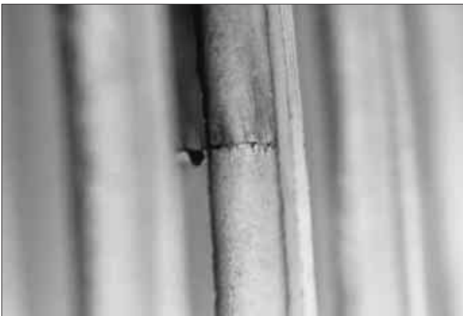
Figure 2. Crack across weld in spiral heat exchanger.
