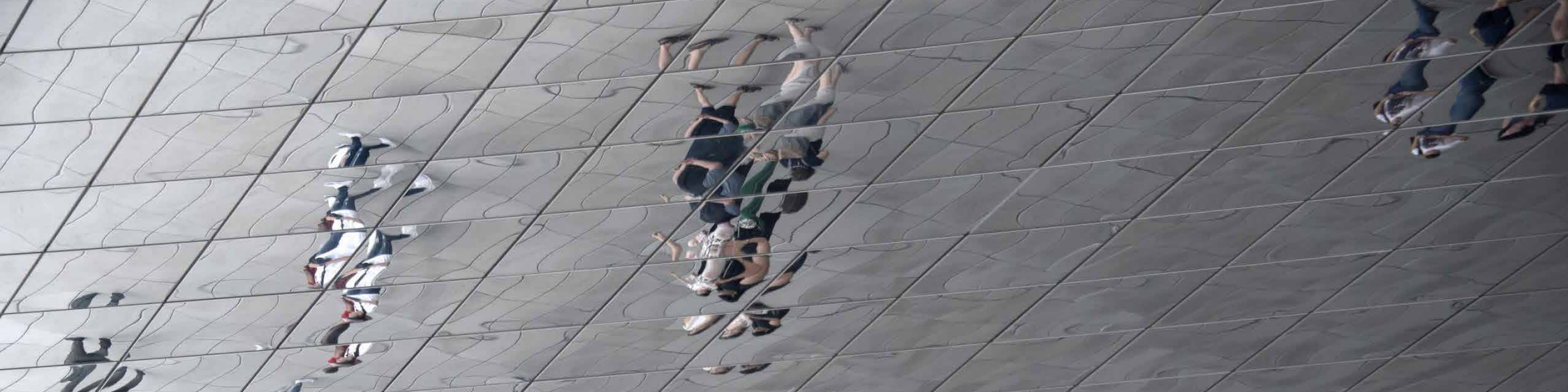
Fig. 3. The ceiling of the Porsche Museum lobby in Stuttgart, Germany is clad with mirror polished Supra 316L/4404 stainless steel produced by Outokumpu.
