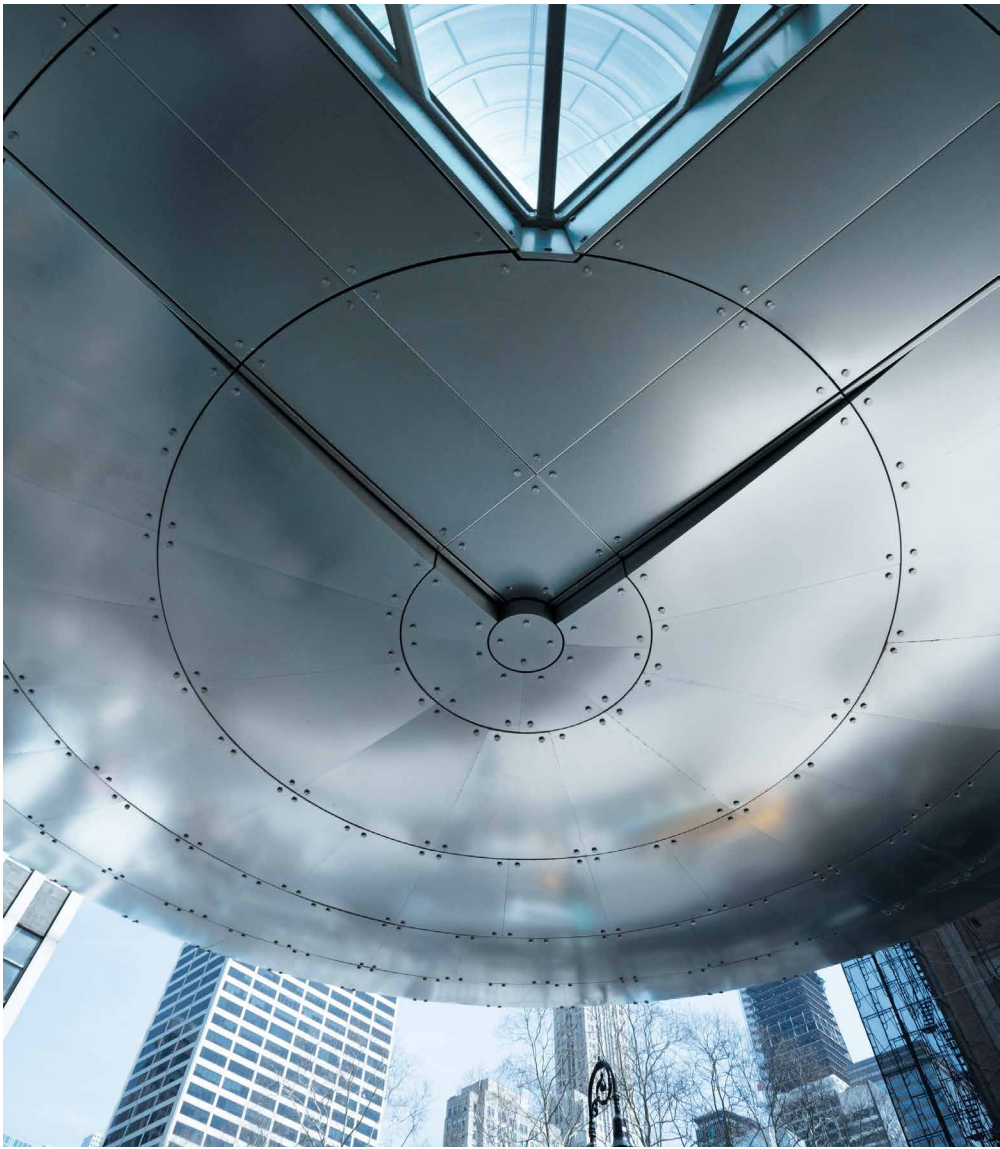
Fig. 1. A detail of the entrance to 7 Bryant Park, New York which is clad with Outokumpu Deco Linen.
