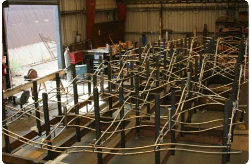
The undulating frame of the 38' x 19' sculpture at the Smithsonian's new Star Spangled Banner exhibit is made entirely of Outokumpu's LDX 2101® stainless bar. The sculpture (shown here mid-fabrication) was fabricated at TriPyramid Structures, Inc. Photo courtesy of TriPyramid Structures, Inc.
