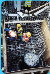
LDX 2101® can be used in rebar applications. Photo courtesy of Anaco Trading Ltd. Australia
