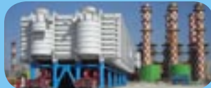
SIDEM and Outokumpu first partnered in 2006, to build the Al Hidd desalination plant in Bahrain.
