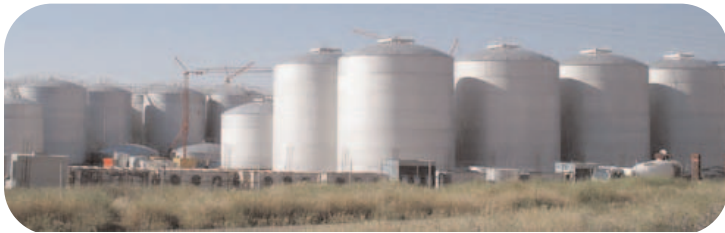
This pressure vessel for Smurfit Kappa Kraftliner Piteå is made entirely out of LDX 2101®.
