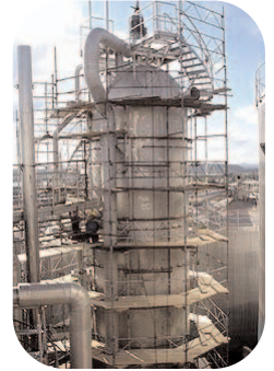
Wine is now being stored in tanks built with LDX 2101®.
