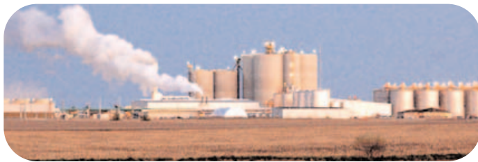
VeraSun Energy in Charles City, Iowa features two ethanol storage tanks and four corn storage tanks.
