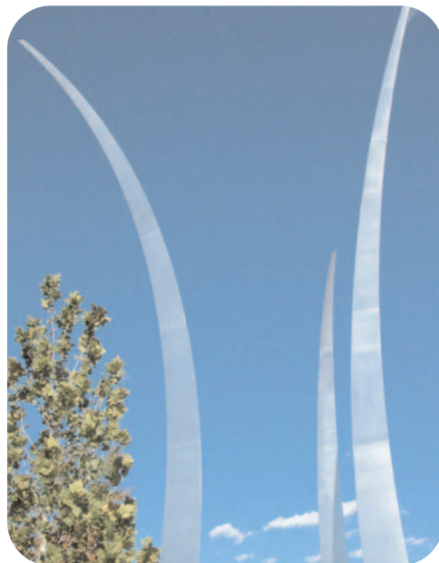
Grade ASTM 316L was used in the construction of the Air Force Memorial. Photo by Catherine Houska, TMR Stainless
